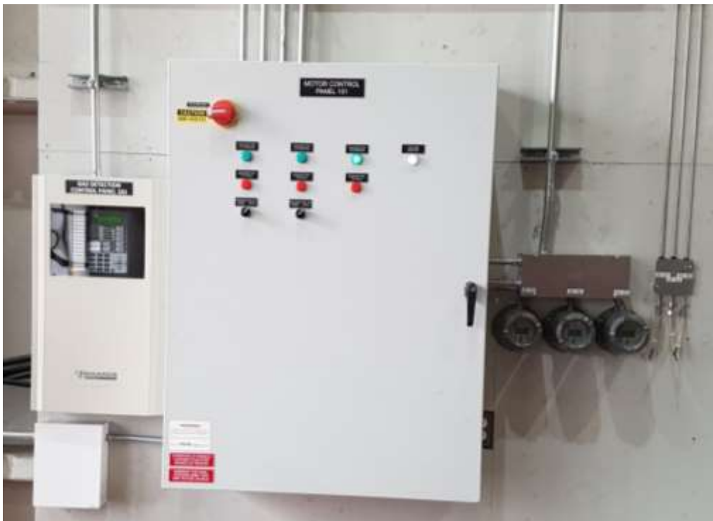
Figure 7.4 – gas safety control system
