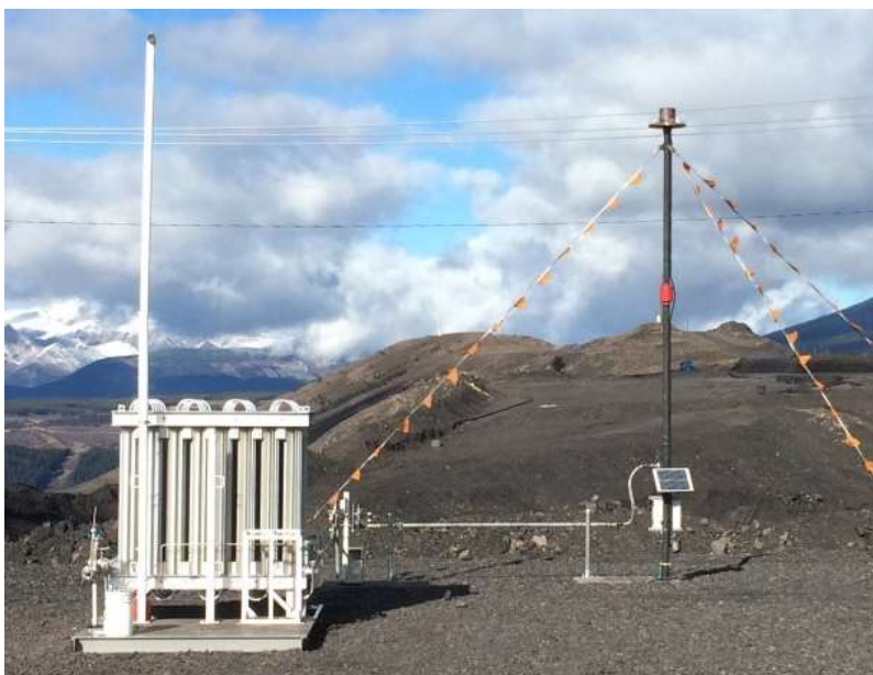
Figure 9.5 – LNG container de-fuel vaporizer and flare
