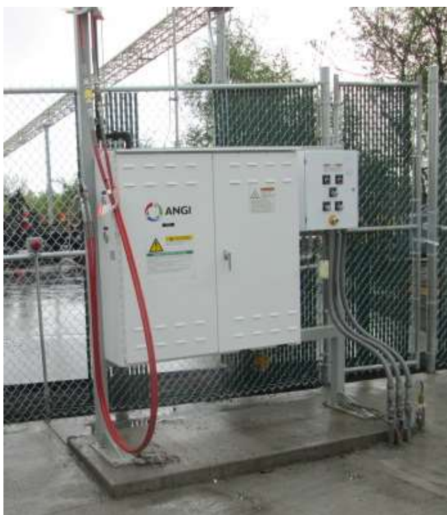
Figure 9.2 – De-fuel panel and post
