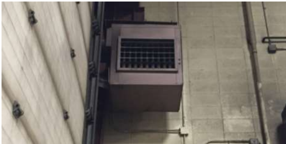
Figure 6.4 – Fired Unit Heater
