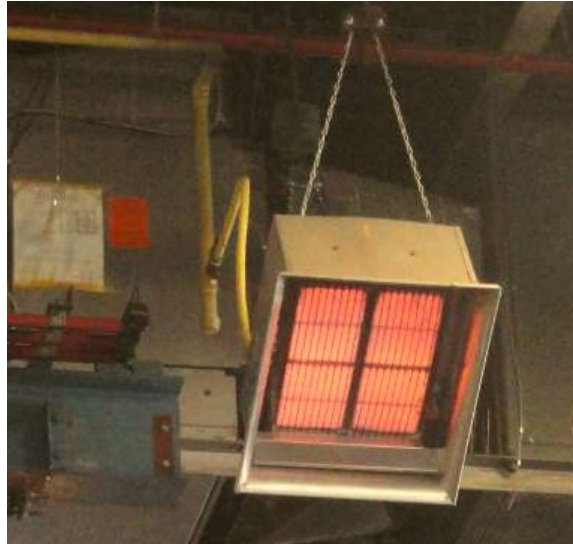
Figure 6.3 – natural gas catalytic heater
