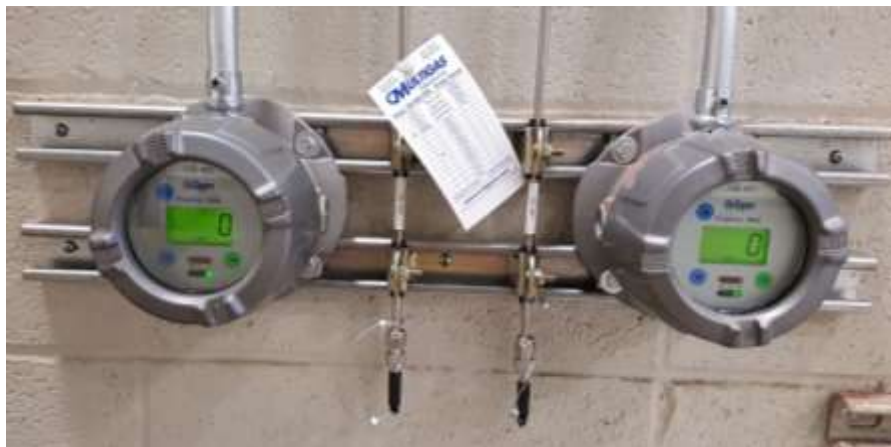
Figure 7.3 – gas sensor calibration tubing
