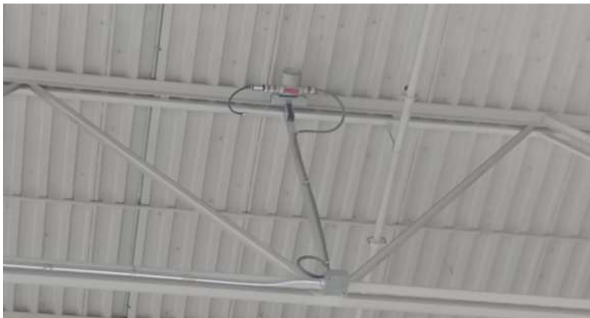
Figure 7.1 – fixed point gas sensor
