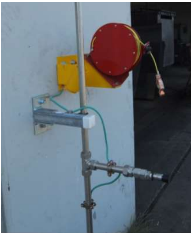
Figure 9.3 – de-fuel vent systems – no hose shown
