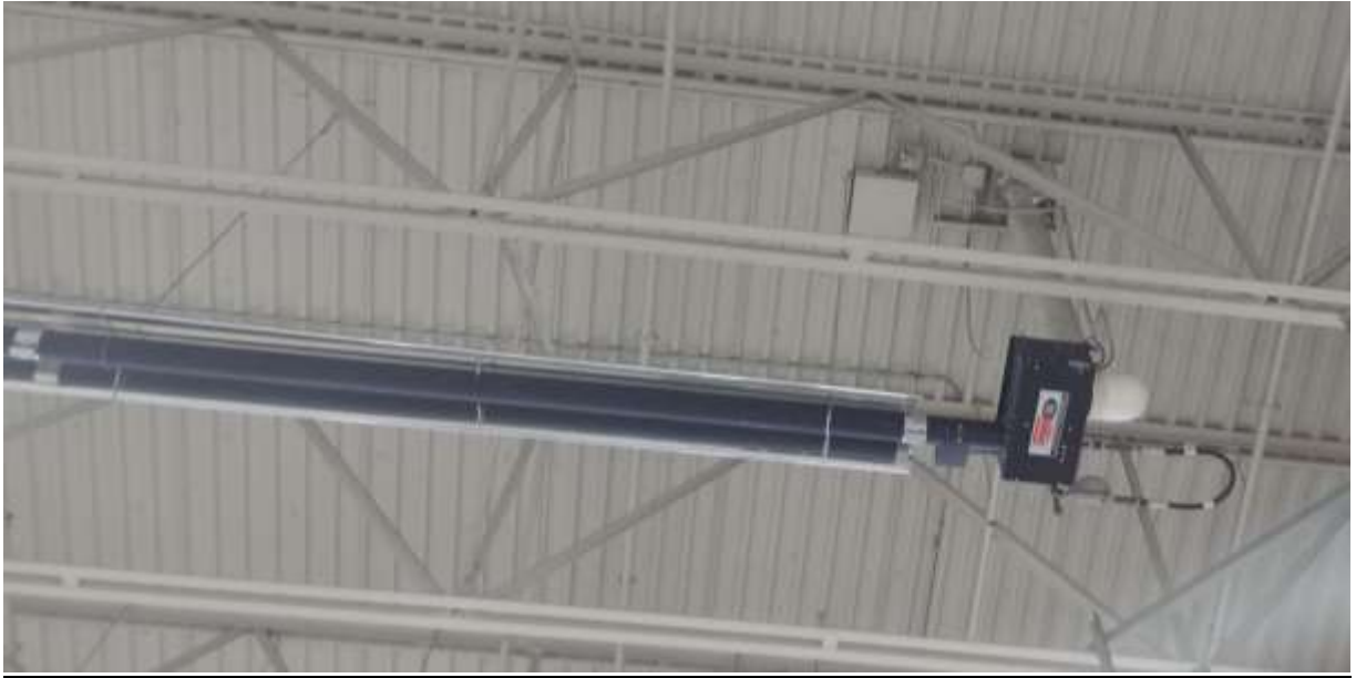
Figure 6.1 – low intensity discrete radiant tube heater
