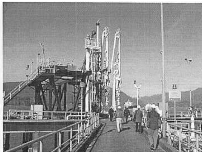
Exhibit 9. The Dock Is Equipped With H 2 S Scrubbers (Left) And Oil Loading Arms (Right)
