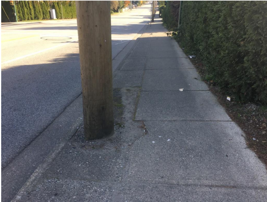
Figure 23 - Example of Sidewalk Out of Elevation (settled patch around pole)
