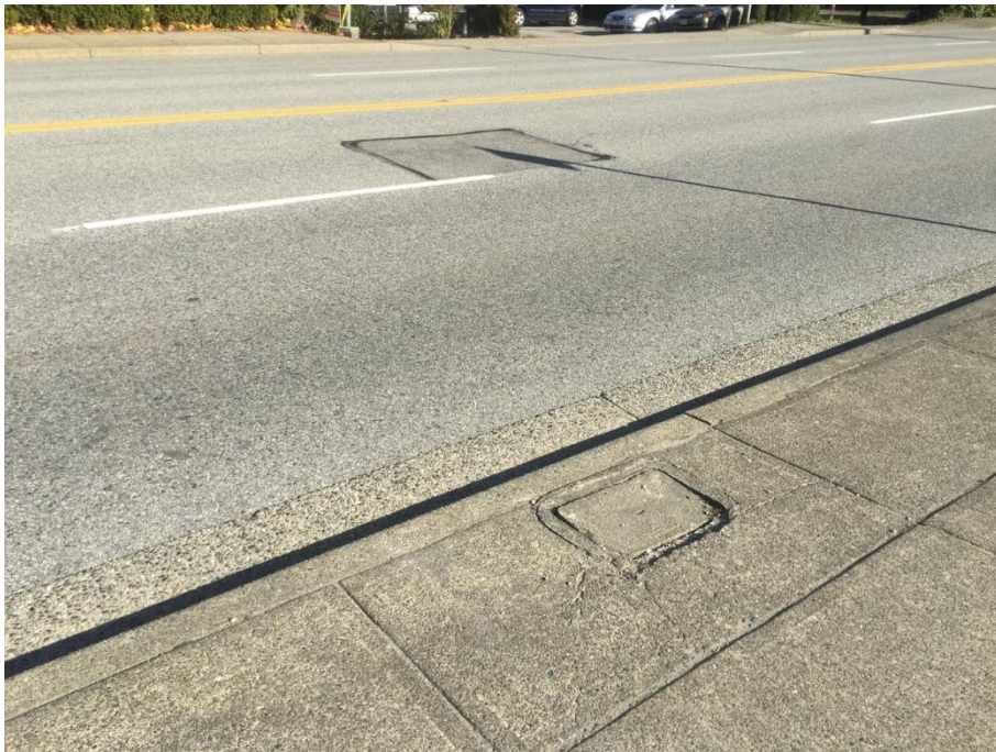
Figure 27 - Example of Observation – Junction / Utility Box Lid Damaged / Settled
