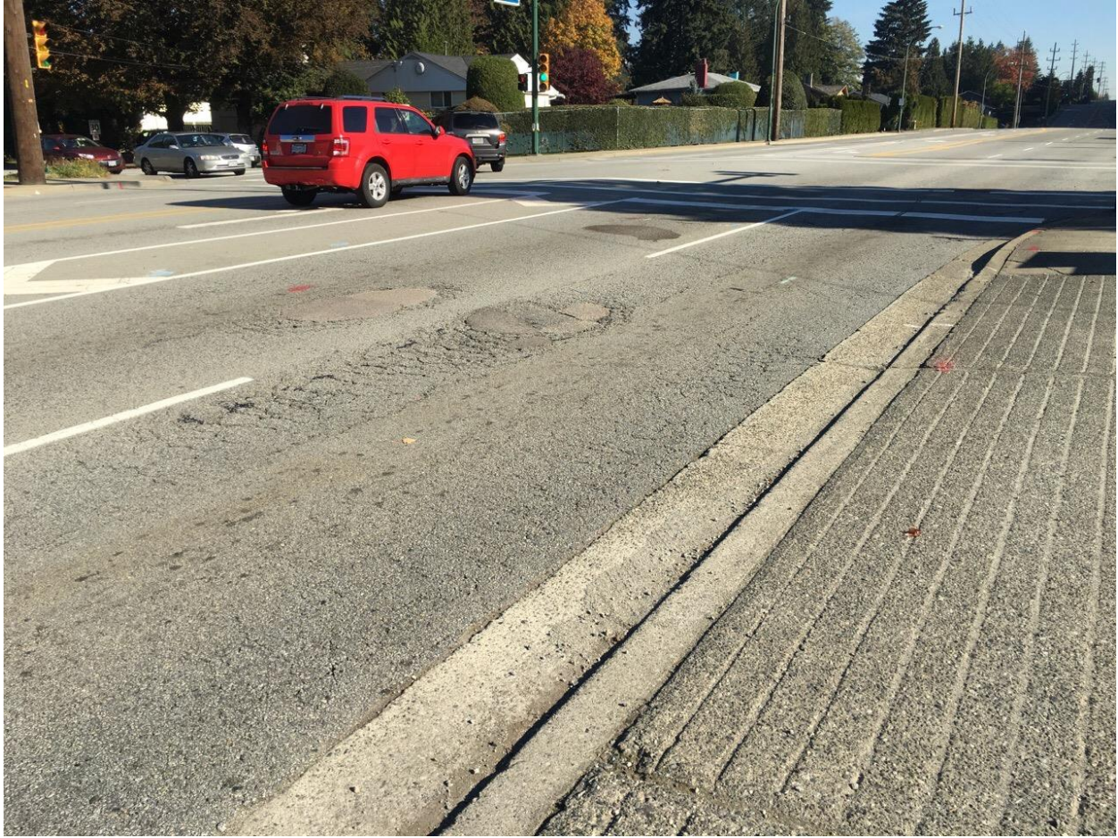
Figure 18 - Example of Alligator Cracking at Thermal St
