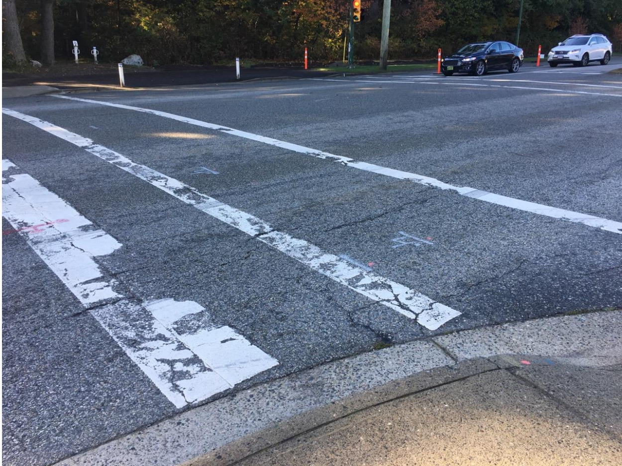
Figure 20 - Example of Alligator Cracking at Baker St
