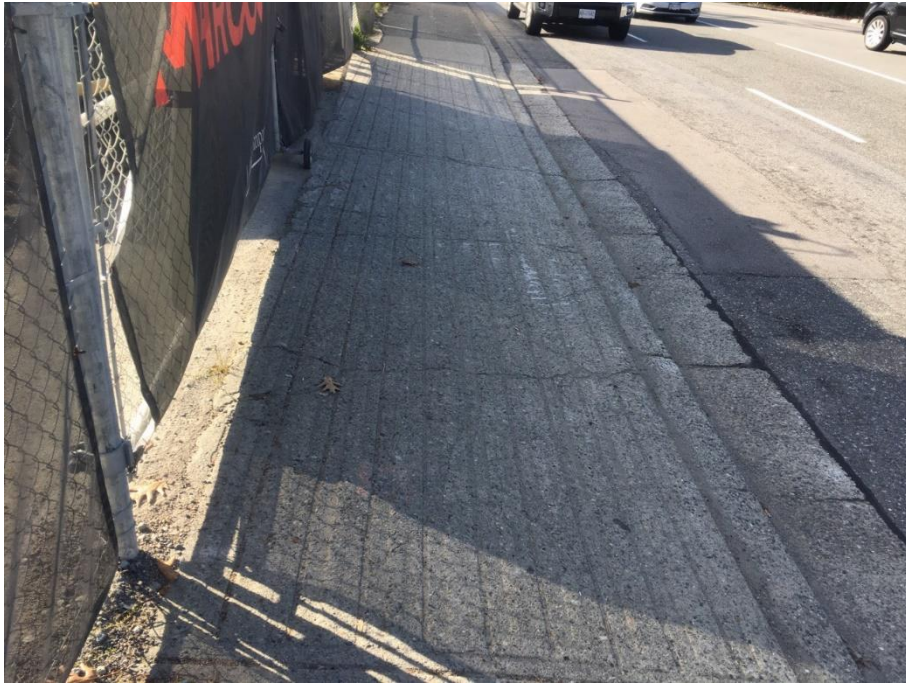
Figure 24 - Example of Sidewalk Cracking - High (driveway crossing next to construction site)
