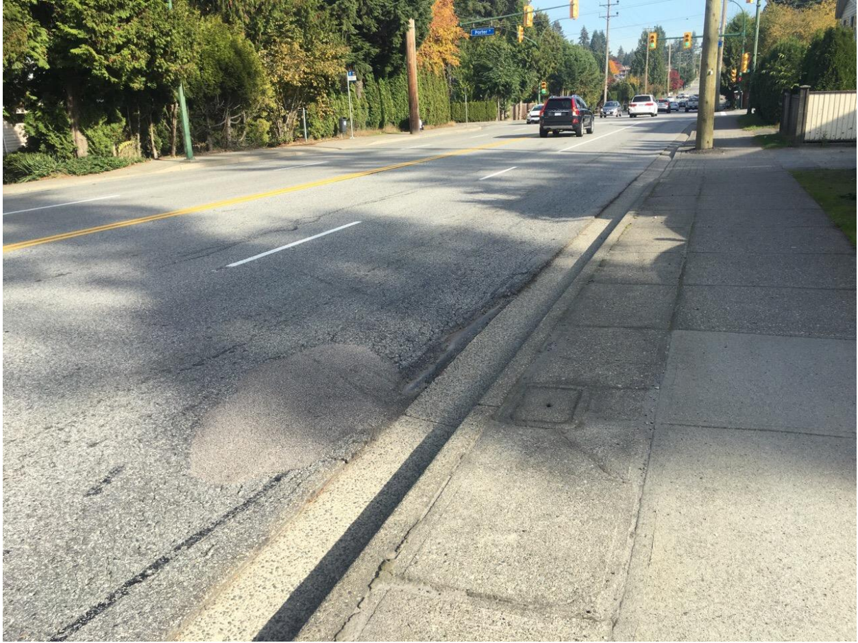
Figure 10 - Example of Alligator Cracking - Near Porter St
