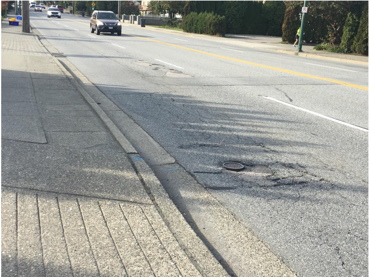
Figure 11 - Alligator Cracking and Patching Near Lillian St
