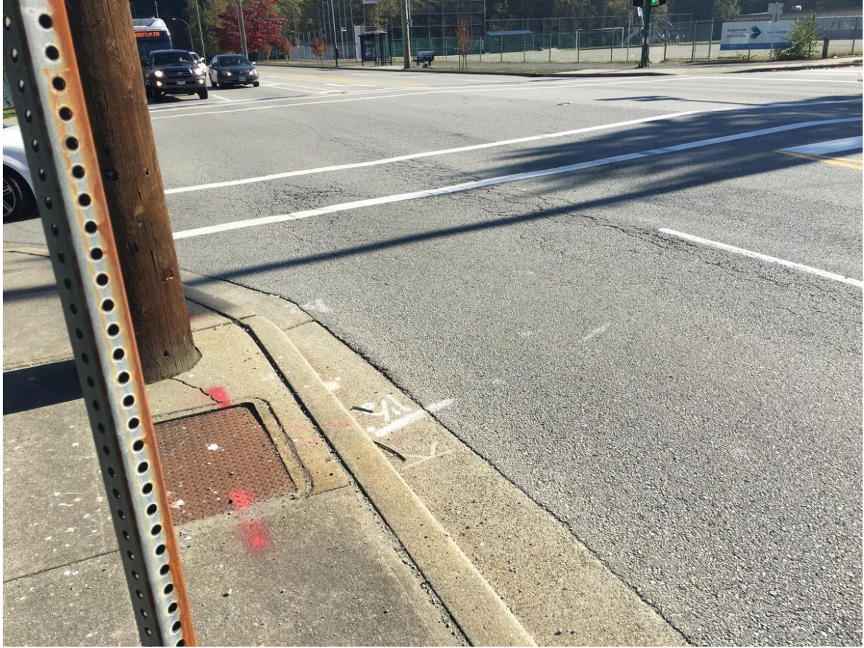
Figure 19 - Example of Alligator Cracking at Thermal St
