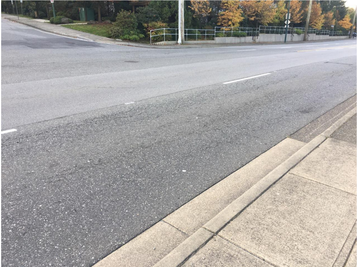
Figure 5 - Example of Alligator Cracking – North to Robinson
