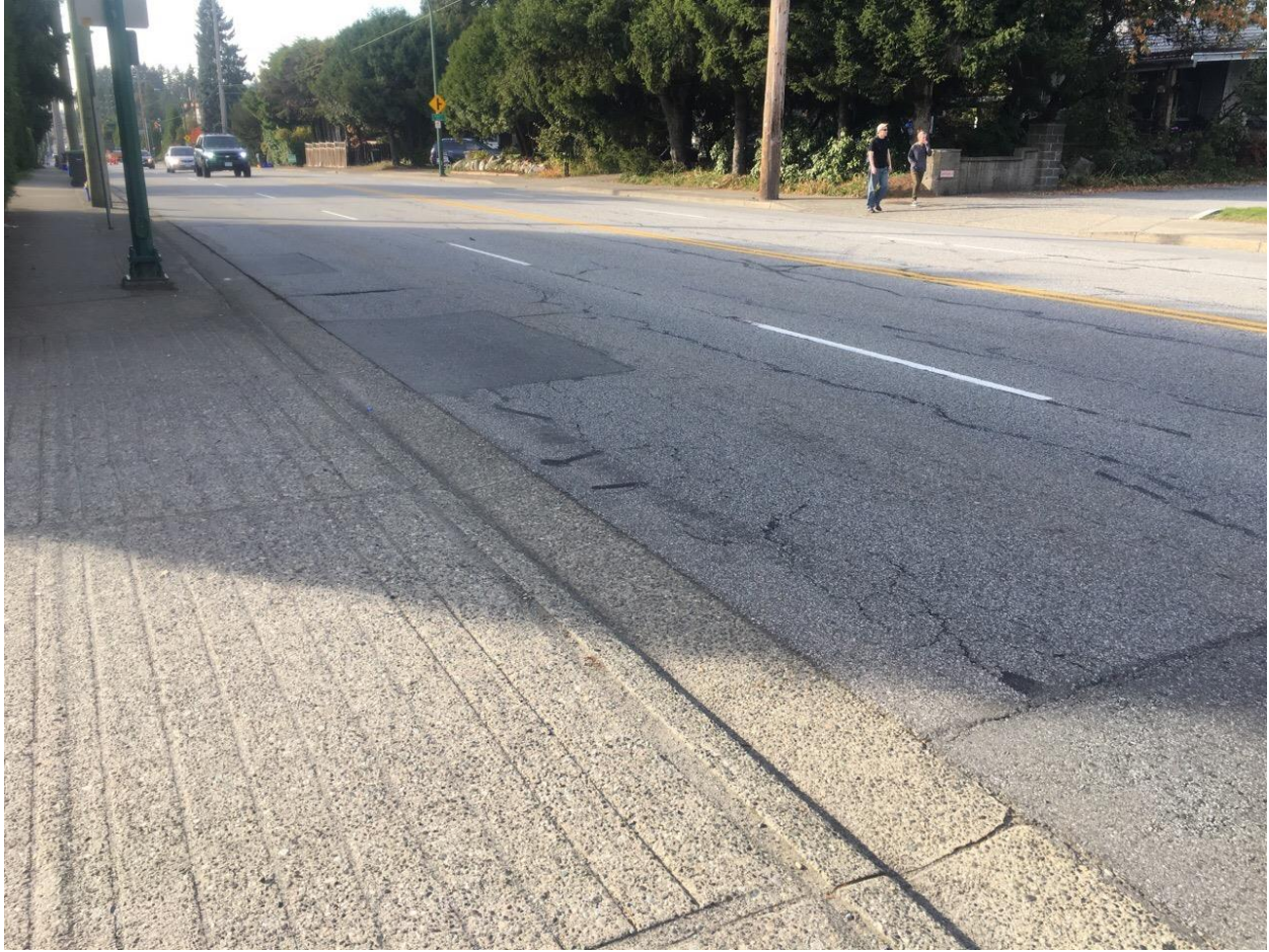
Figure 13 - Example of Alligator Cracking Near Crestwood Dr
