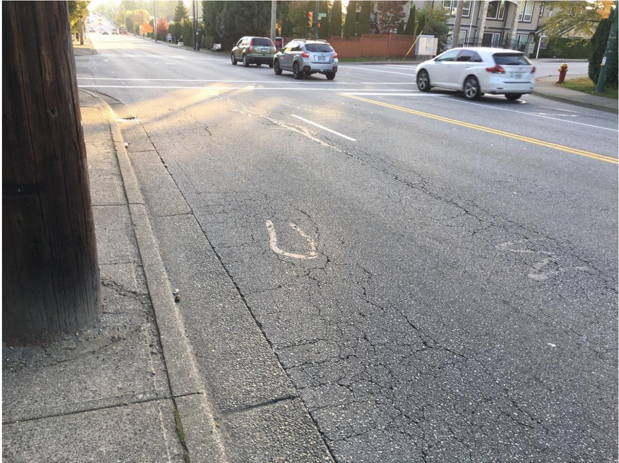
Figure 8 – Example of Alligator Cracking – Near Blue Mountain St
