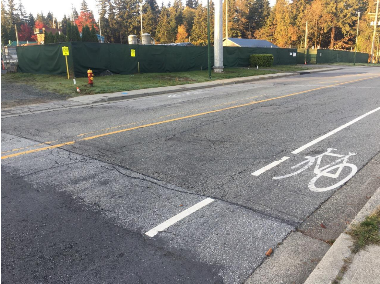
Figure 22 - Example of Alligator Cracking West of Pinnacle St
