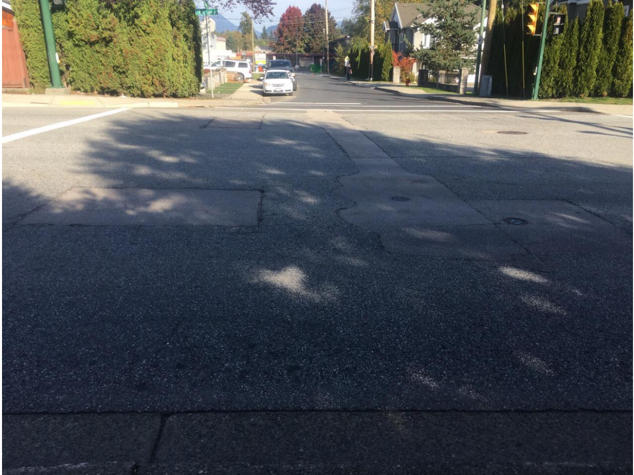
Figure 7 - Example of Patching at Banting St
