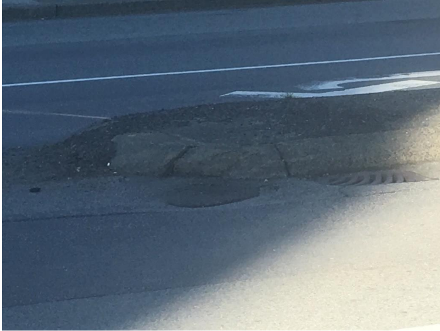
Figure 26 - Example of a Broken Median
