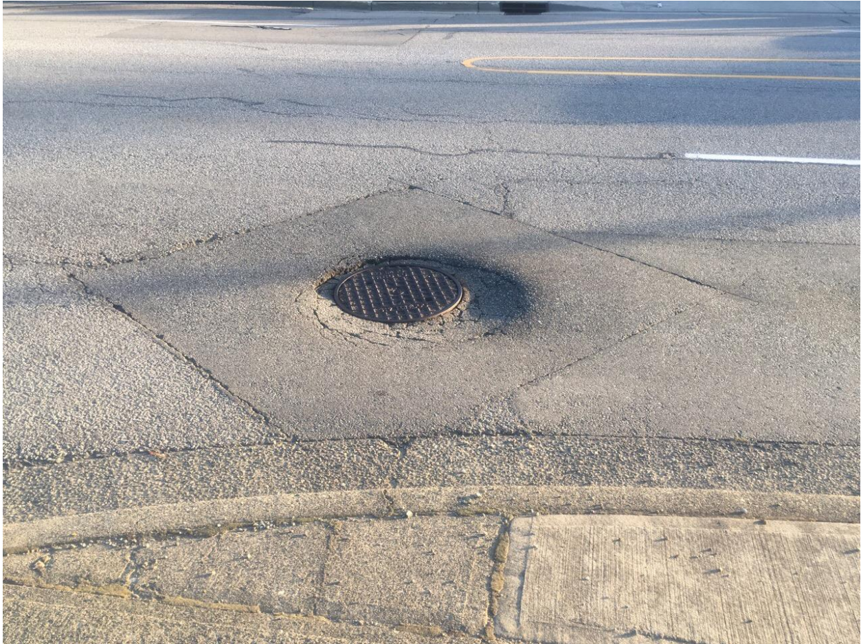
Figure 12 - Example of Patching at Regent St
