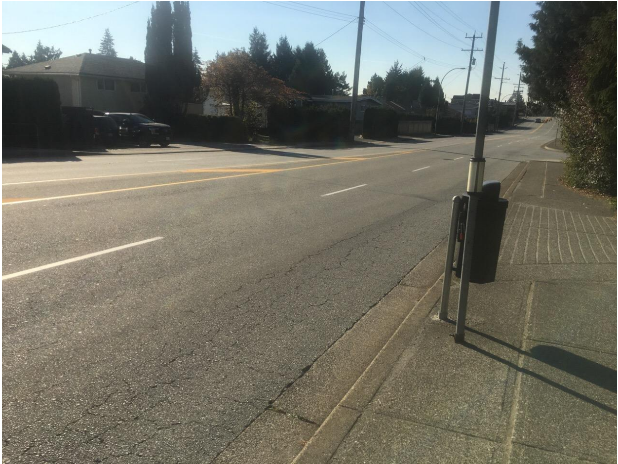
Figure 17 - Example of Alligator Cracking Near St Laurence St
