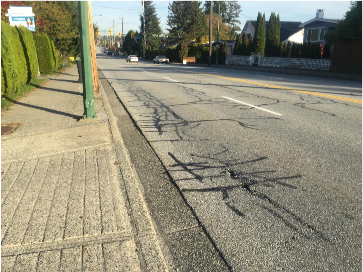
Figure 14 - Example of Alligator Cracking Near Wasco St
