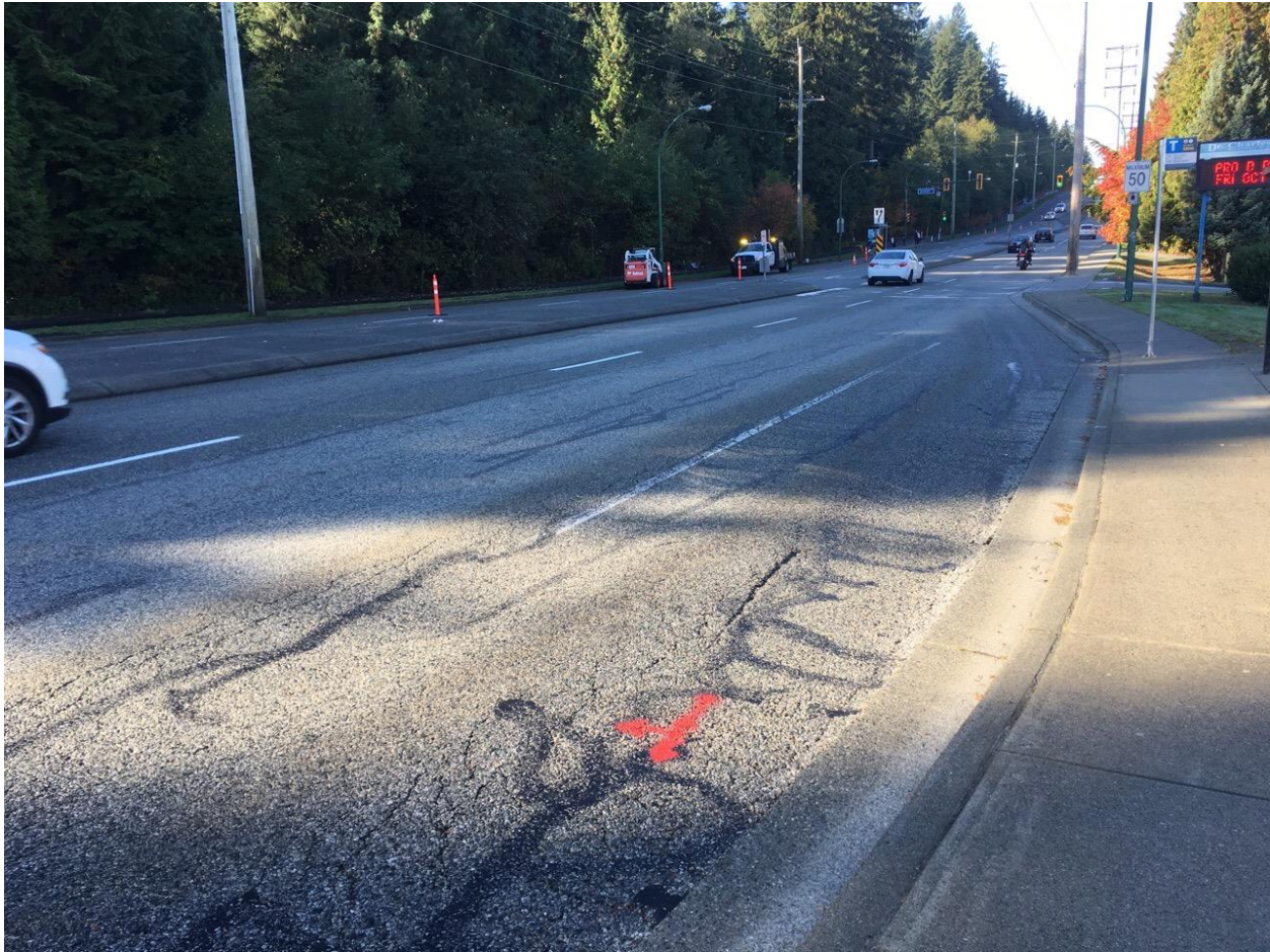
Figure 21 - Example of Alligator Cracking and Distortions East of Baker at Bus Stop
