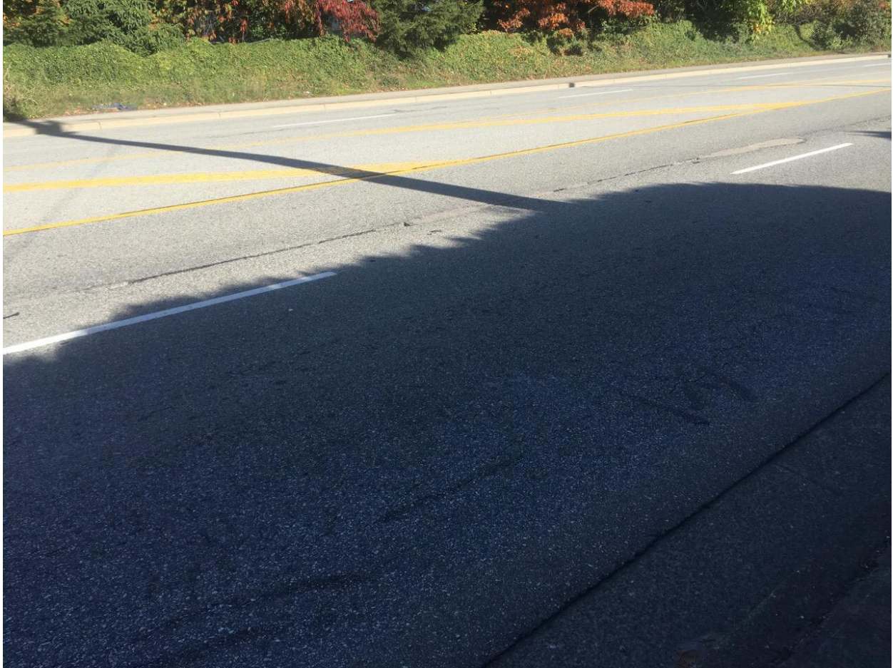
Figure 9 - Example of Linear Cracking and Alligator Cracking Near Blue Mountain St
