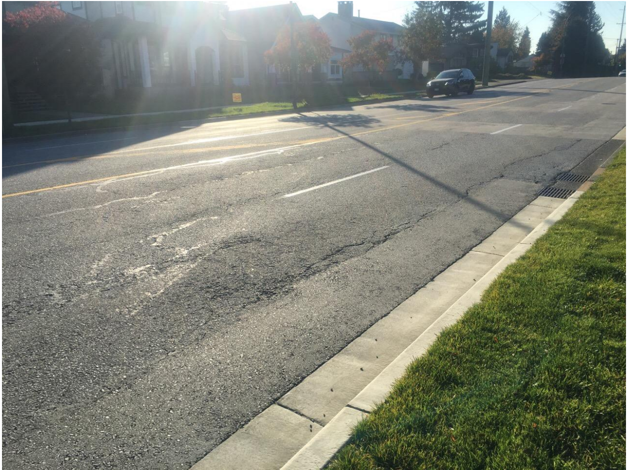
Figure 15 - Example of Distortion and Cracking Near Poirier St
