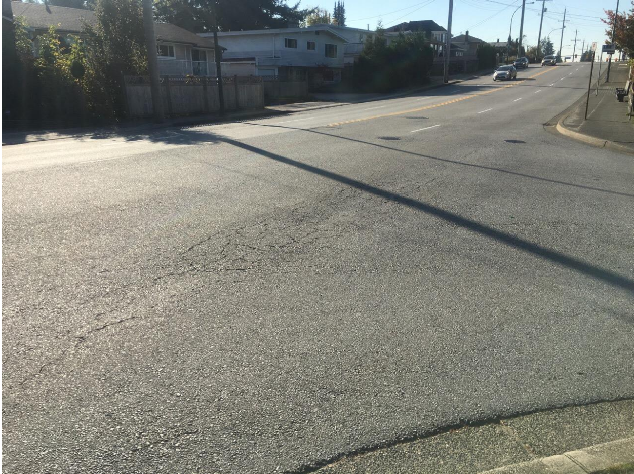
Figure 16 - Example of Alligator Cracking at Prospect St
