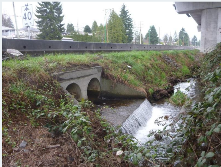
PHOTO 17: VIEW OF THE OUTLET OF THE TWIN CULVERTS LOCATED ALONG THE FELL AVE ALIGNMENT, FLOW FROM THIS POINT IS CONVEYED TO THE EAST ALONG THE SOUTHERN SHOULDER OF LOUGHEED HWY. PHOTO FACING EAST (DOWNSTREAM), TAKEN ON MARCH 19, 2015.
