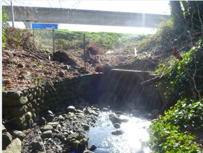
PHOTO 22: VIEW OF THE 1200 MM CONCRETE CULVERT CONVEYING FLOW FROM POLLYWOG CREEK TO THE SOUTH ACROSS LOUGHEED HWY. PHOTO FACING SOUTH (DOWNSTREAM), TAKEN ON FEBRUARY 27, 2015.
