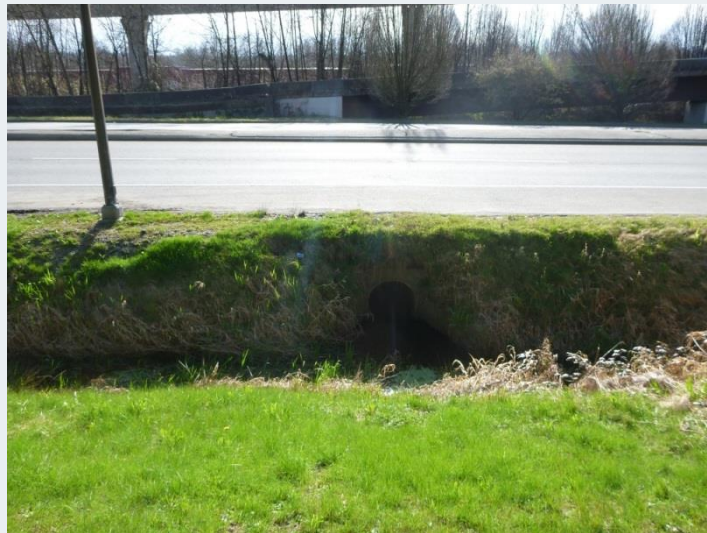
PHOTO 21: VIEW OF THE CULVERT LOCATED APPROXIMATELY 80 M TO THE WEST OF SPERLING AVE, FLOW FROM THIS POINT IS CONVEYED SOUTH TO SPARTAN CREEK. PHOTO FACING SOUTH (DOWNSTREAM), TAKEN ON FEBRUARY 27, 2015.
