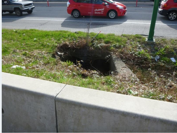
PHOTO 16: VIEW OF THE TWIN ROAD CROSSING CULVERTS LOCATED AT THE FELL AVE ALIGNMENT. FLOW FROM THIS POINT IS CONVEYED TO THE SOUTH TO THE SOUTHERN SHOULDER OF LOUGHEED HWY. PHOTO FACING SOUTH (DOWNSTREAM), TAKEN ON FEBRUARY 27, 2015.
