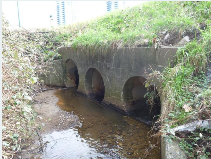
PHOTO 9: BEECHER CREEK IS CONVEYED TO THE SOUTH OF LOUGHEED HWY THROUGH THREE CONCRETE CULVERTS. PHOTO FACING DOWNSTREAM (SOUTH), TAKEN ON FEBRUARY 27, 2015.
