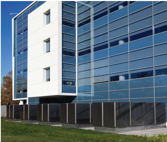
FIGURE 6: Bloom Energy Server Outdoor Installation
