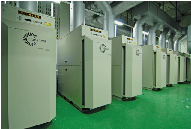
FIGURE 9: Microturbine Installation
