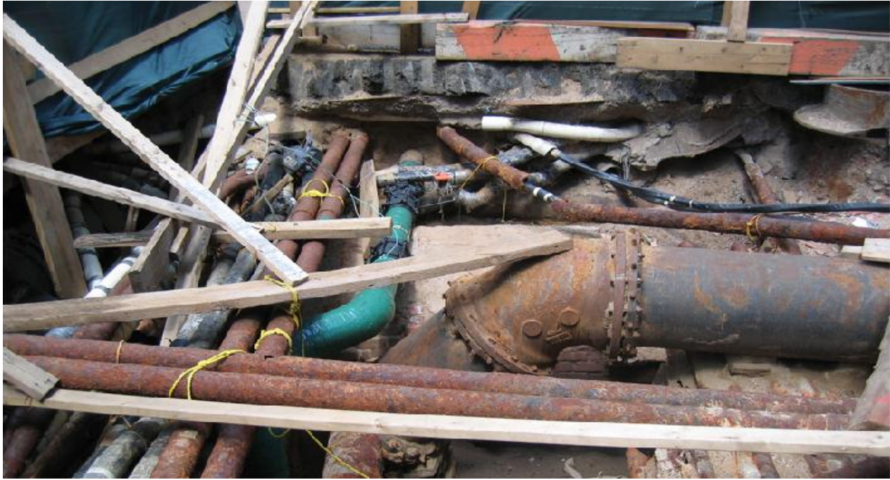
Figure 2 Co-Location of Gas Pipe in an Urban Trench
