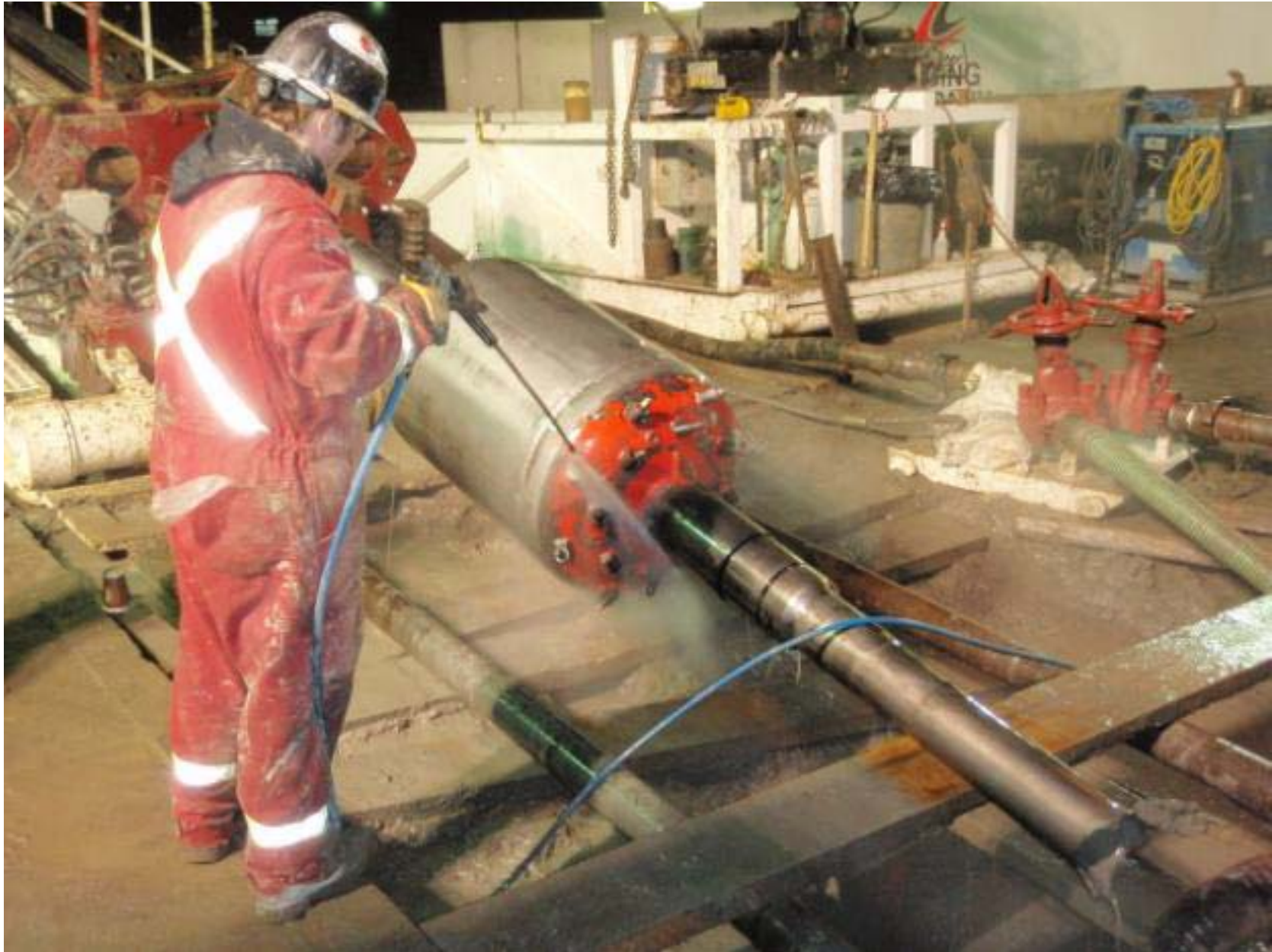
Jan 23, 2010. North side – recovered reamer and North end of HDD drill string. Drill pipe end at lower right was explosively sheared to effect the recovery. 1100 metres of HDD drill string left abandoned beneath Fraser River.
