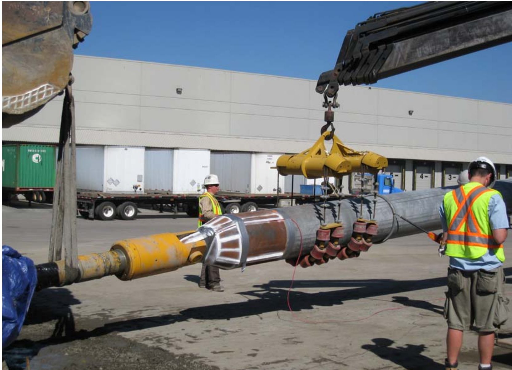
July 24, 2010.. North Side – NPS 24 pullback about to begin. When the pullback was 96% complete, the swivel joint (shown here in-between the grey nylon sling and the pull-head attachment pin) pulled apart.
