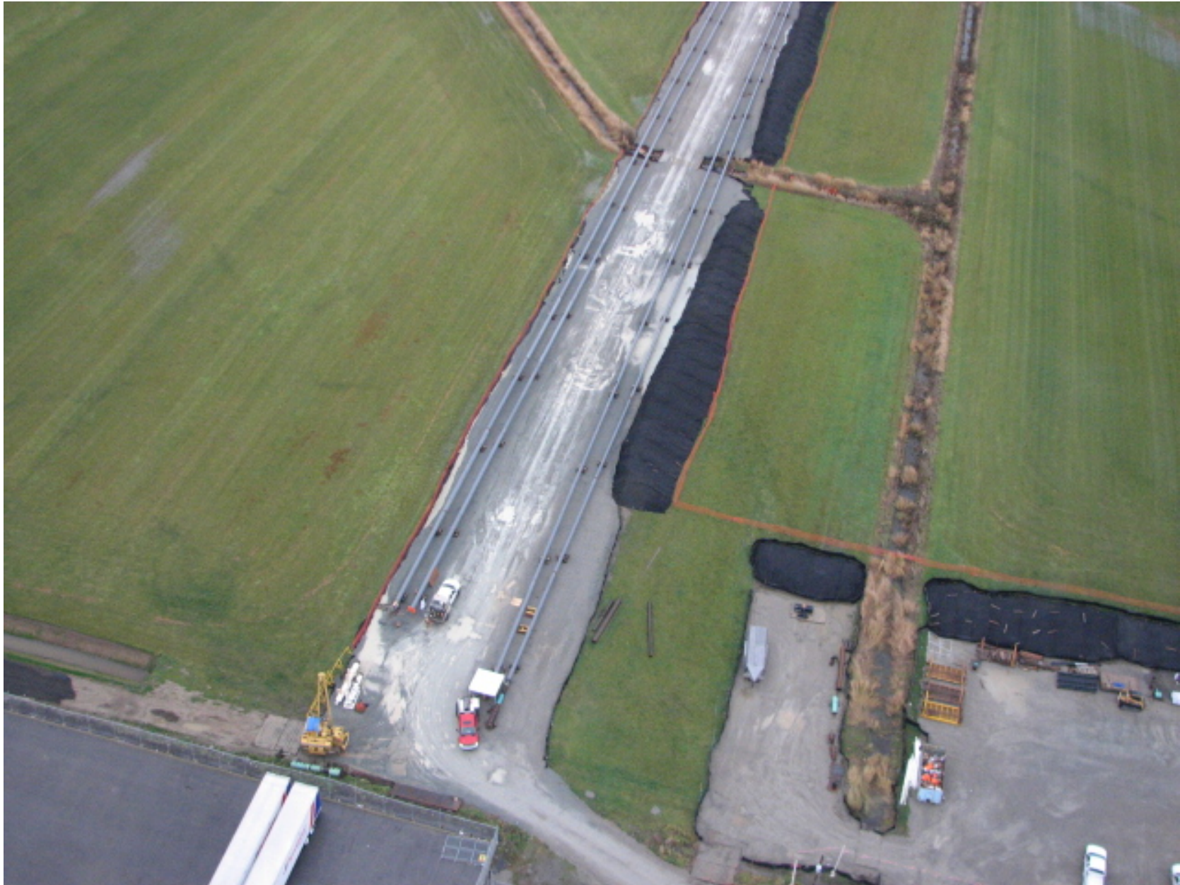
Nov 26, 2009 – Pipe Layup Area showing completion of four HDD Pipe Strings Two NPS 20 and two NPS 24. Each string is 800m long.
