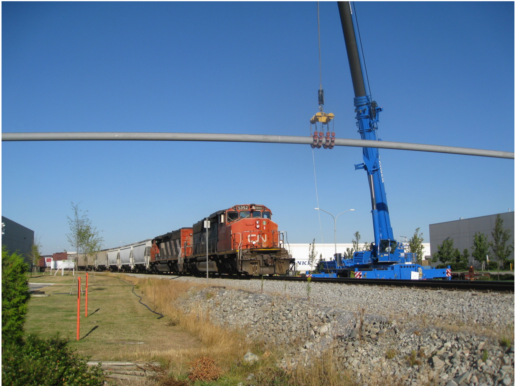
July 24, 2010. North Side, showing NPS 24 pullback underway, traversing active CNR spur line.
