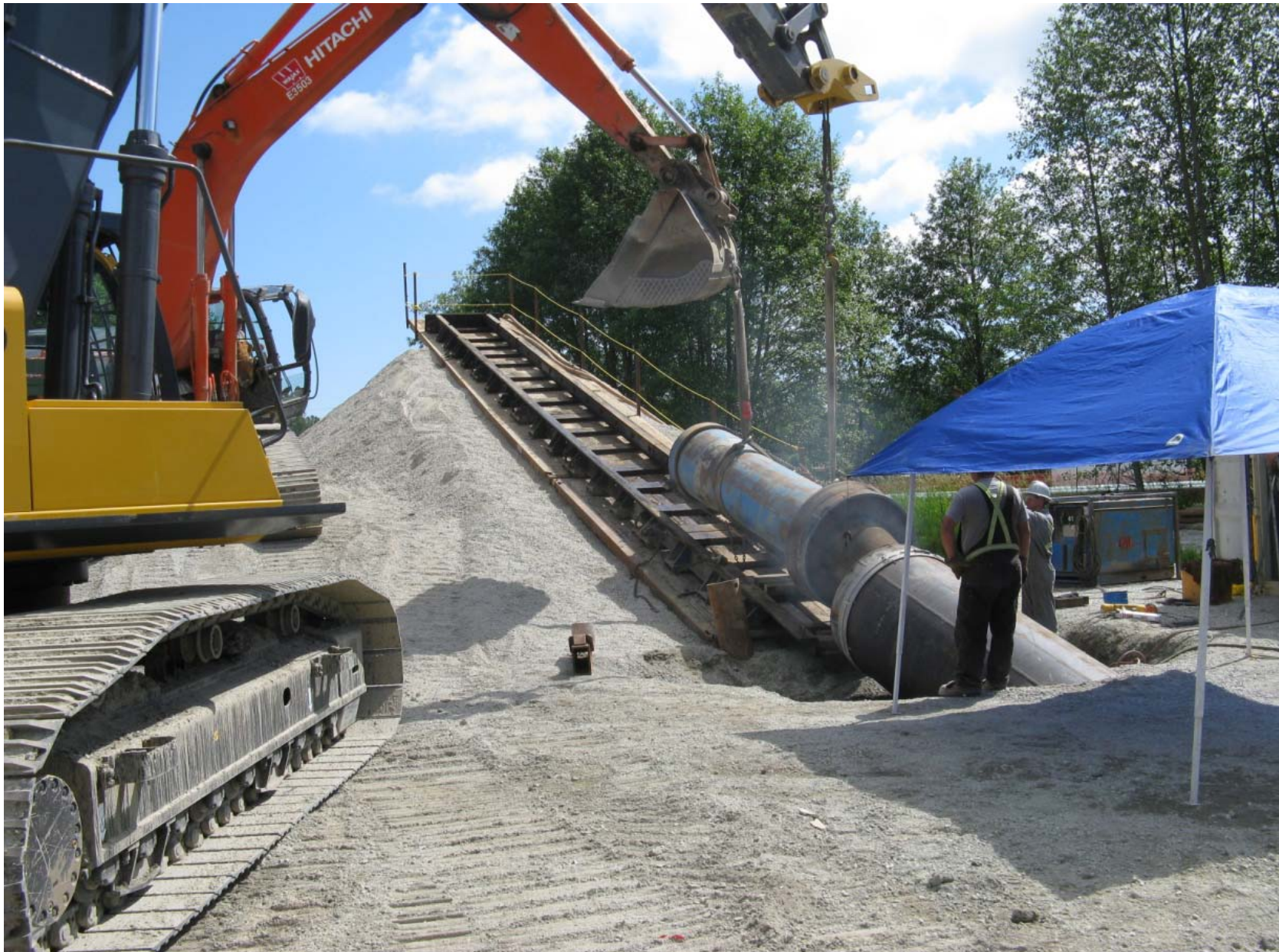
June 13, 2010. New South Side HDD entry casing for re-designed NPS 20 HDD alignment. Removal of hydraulic hammer before positioning next segment of casing.
