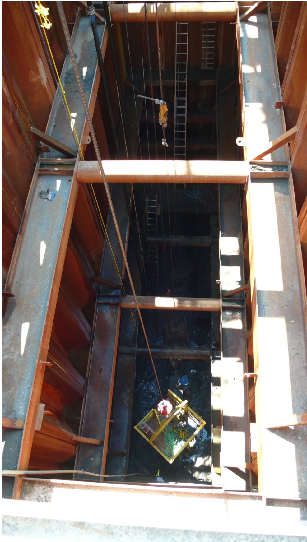
South Side – Completed Cofferdam. Aug 4, 2011
