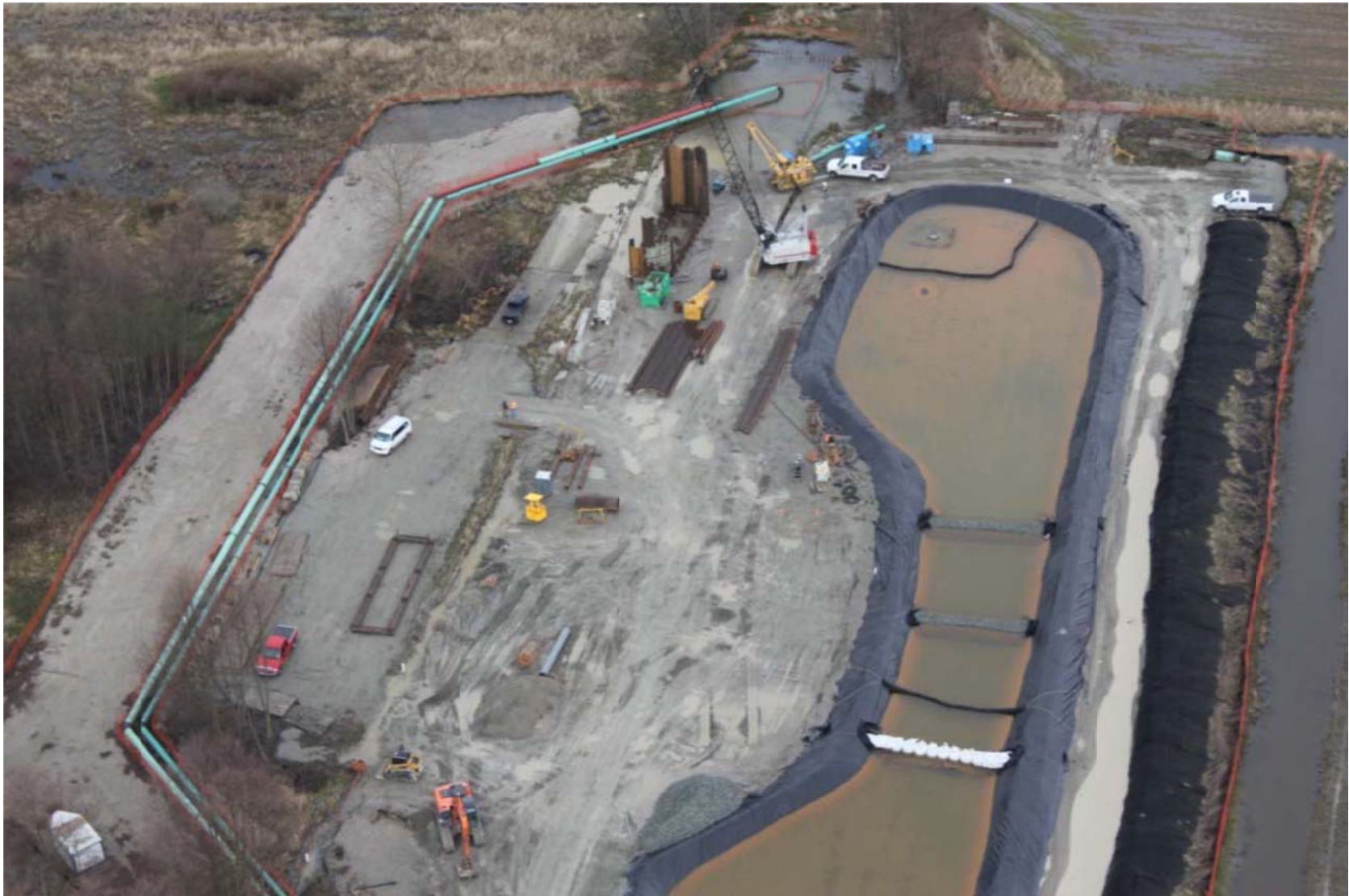
March 23, 2011. Aerial view of the South side Work-site during sheet piling installation. Bypass pipelines at left; pond at right converted for groundwater treatment.
