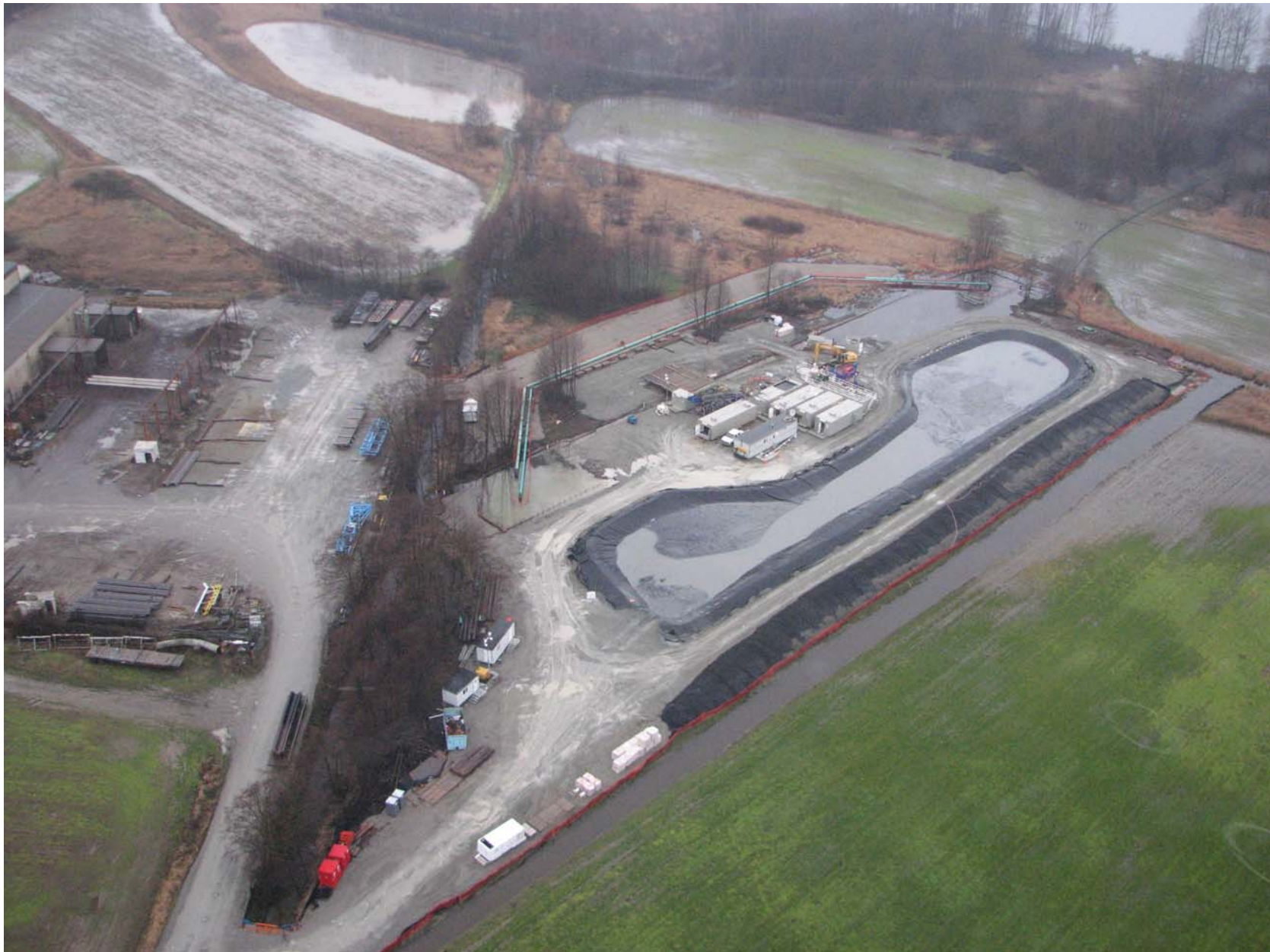
Dec 30, 2009. South side HDD work pad. Showing bypass pipelines and containment pond for drill cuttings.
