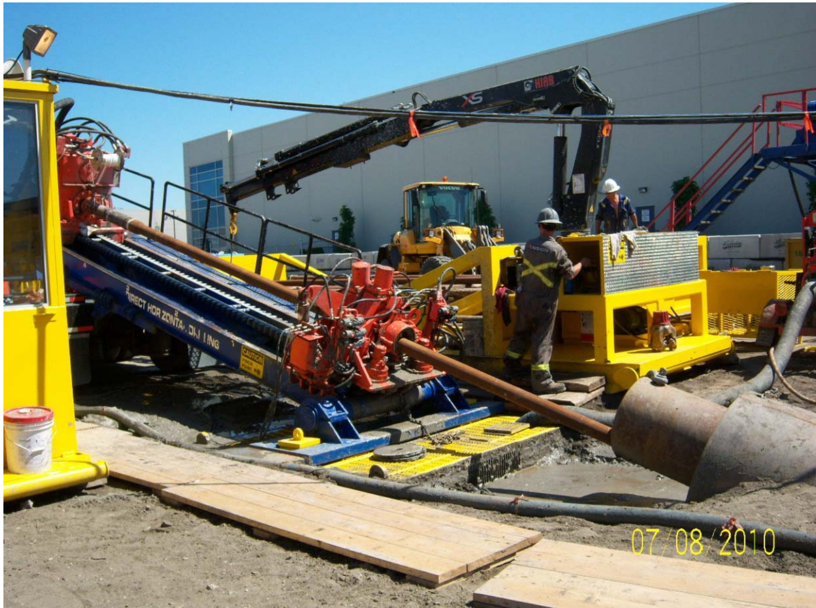
July 8, 2010. North Side - Drilling of intersect pilot hole for NPS 24.
