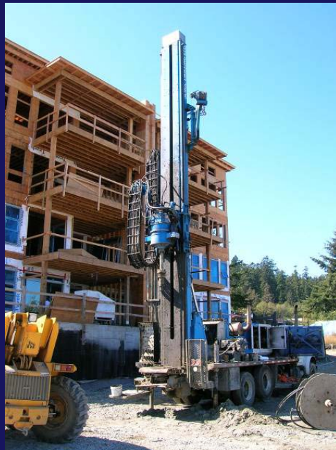
Geothermal drilling
