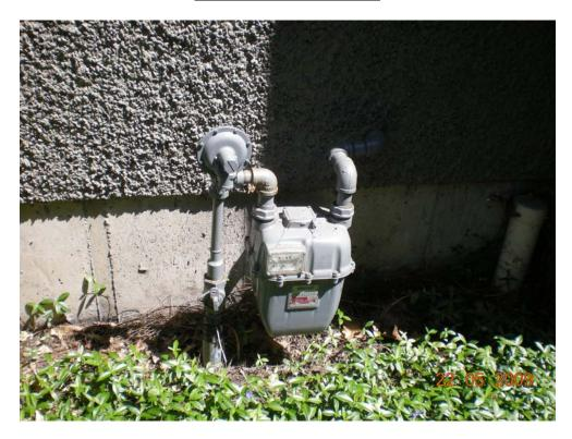
**Upgraded Gas Meter Set with Over Pressure Cut Off (OPCO) Regulator**
