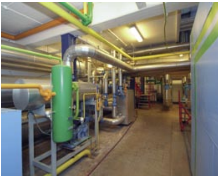
Part of the deairrator system, the pump and the heat exchanger
