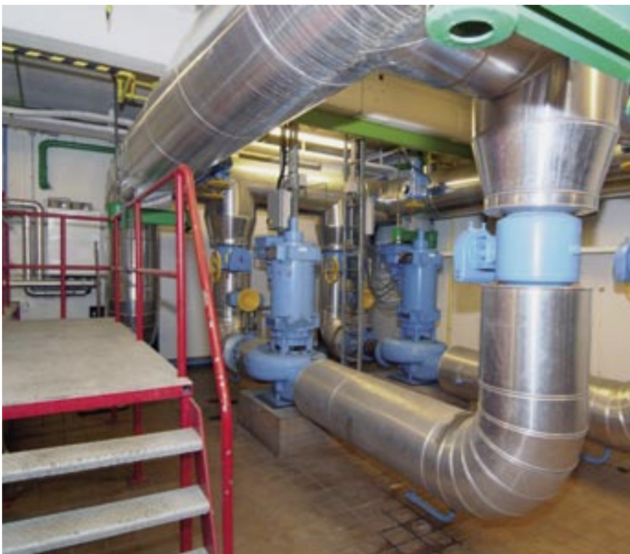
Circulation pumps from VEKS, to the Albertslund 50 MW heat exchanger
