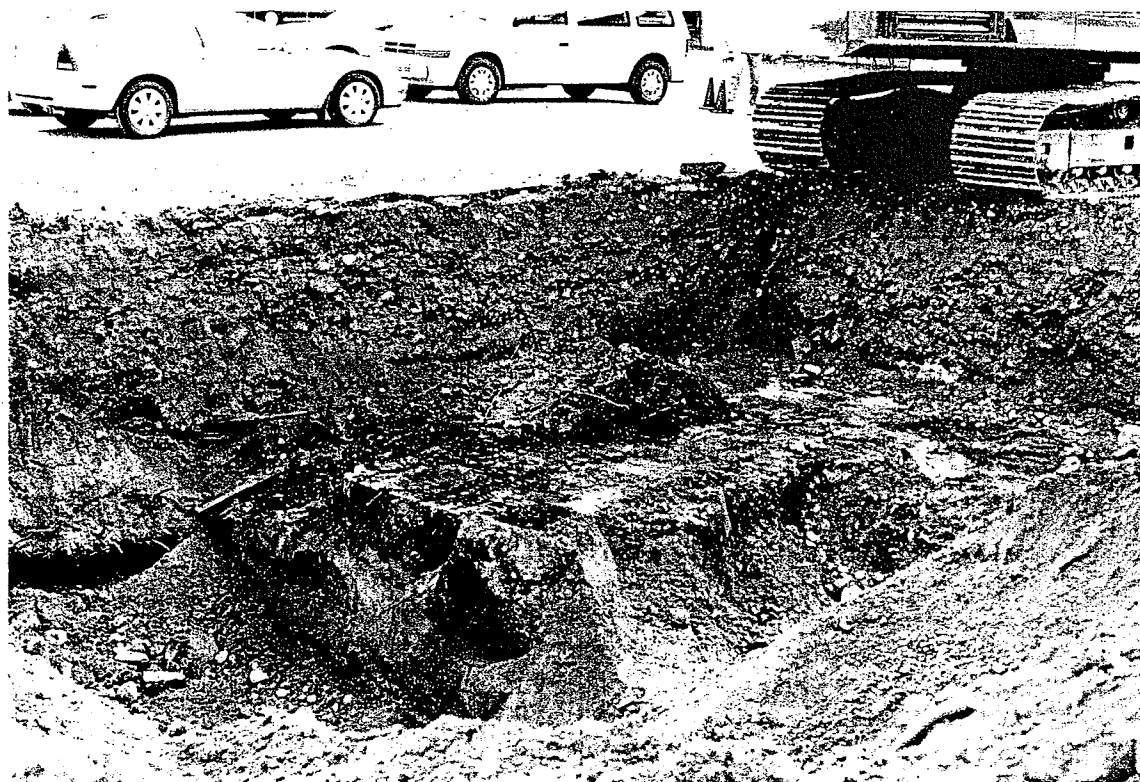
Photo 4: Removal of cover material above peat seam.
