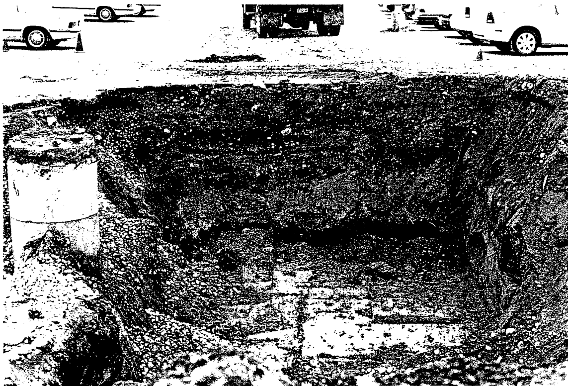
Photo 7: Peat seam pinches out at east side of excavation.
