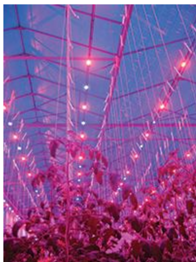
Lemnis LED lights with water cooling in a large-scale trial in tomatoes at Redstar (the Netherlands).
