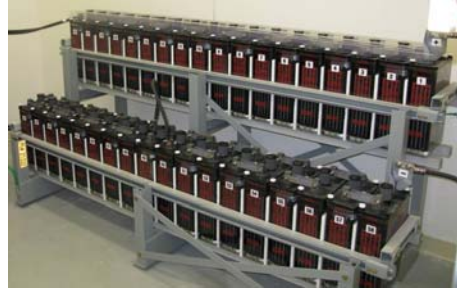
New replacement batteries
