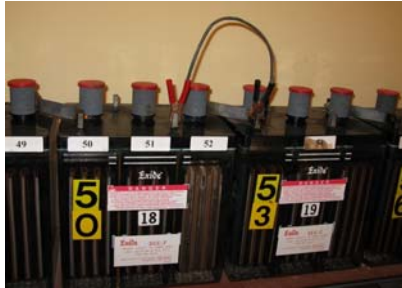
Existing batteries requiring replacement
