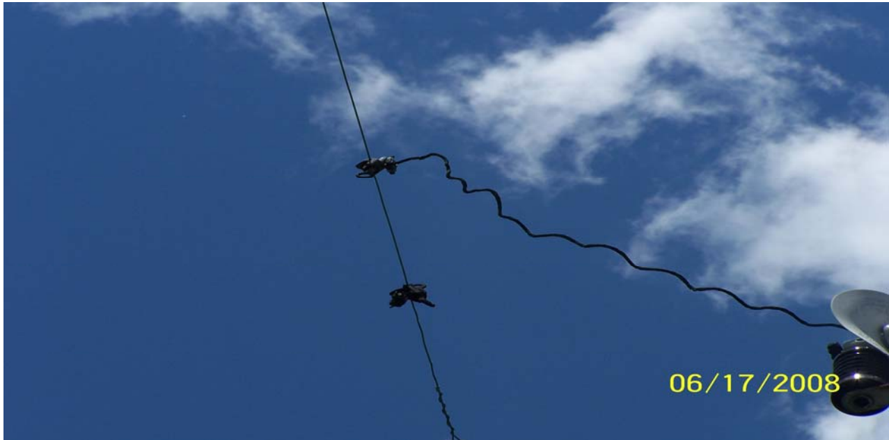
3 Picture 2 4 Hot Tap Connector Left on Conductor
