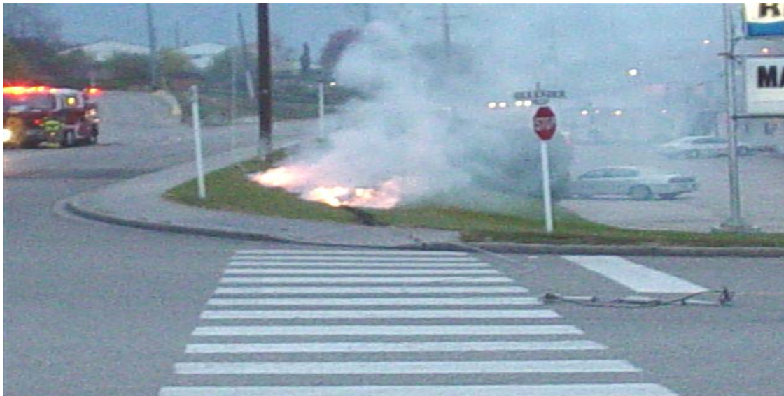
11 Picture 1 12 Energized Power Line on Ground
