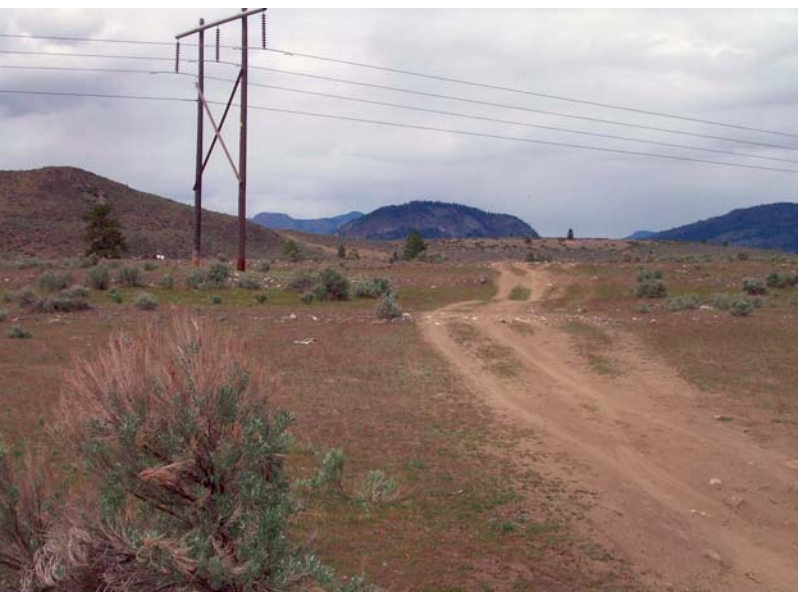
Double steel pole with steel top beam proposed for Oliver to Vaseux transmission line (similar to existing structures shown above)
