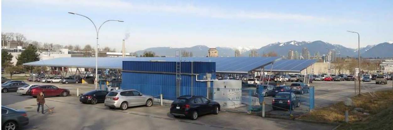
Figure 40: A 500kWh lithium-ion battery system designed and built by Powertech Labs for BCIT's Energy OASIS Project, supporting a 250kW solar canopy over the parking lot, and supplying 2 DCFC and 2 Level 2 EV charging stations.
